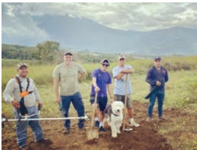
The Official Groundbreaking for Redeemed Steel Guatemala, Ciudad Vieja
